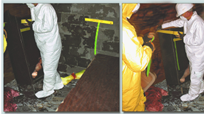
Figure 53. Damaged Building Interior and Marking Methods.
